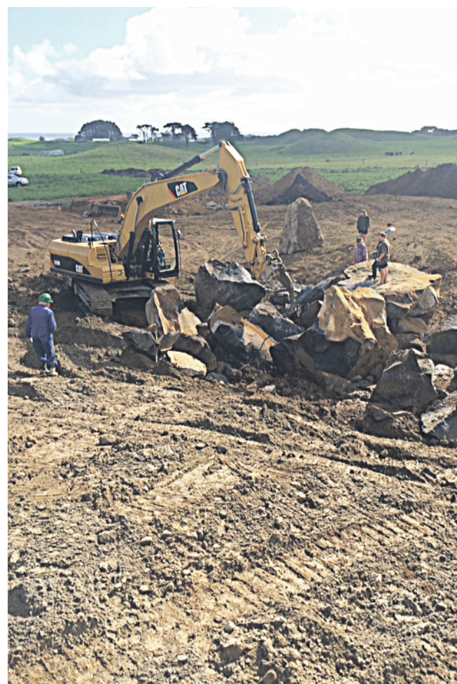
The rock after the explosion, now an easier size for the digger to clean up.
